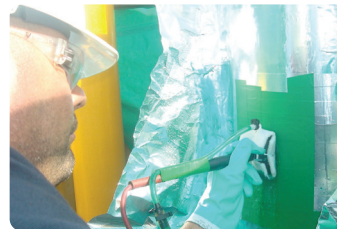
Shaft Repair with AeroNikl® & Cobalt
